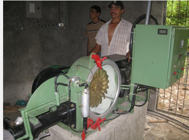
Nicaragua, La Laguna HPP, 60kW, 200l/sec, 47m, 55 fam, 5.5 km grid
