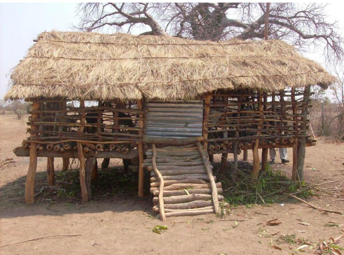
Construction of improved stables
